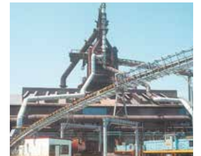
Blast furnace facility
